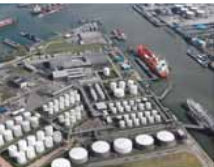
The distribution centre in Rotterdam is perfectly designed for the rapid transshipment of a wide range of tanker types.
